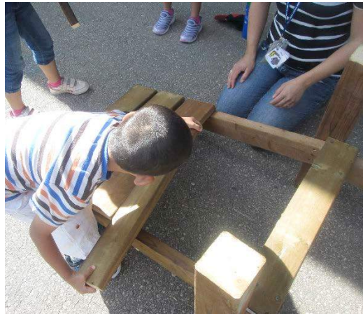
Gavin (4) helping to lay the floor boards on the bridge.
