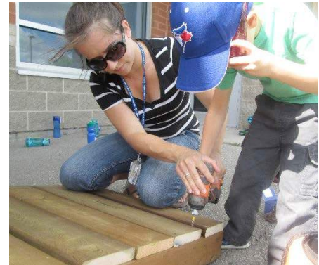
Dylan (5) helping put the last screw in the final floor board of our bridge
